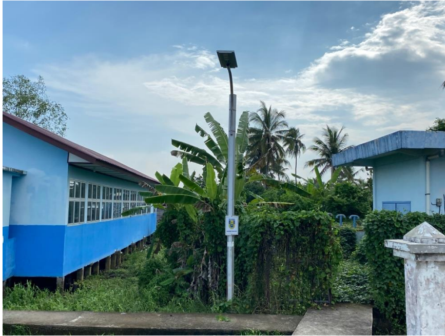
Gambar 3.24 Penambahan Solar Cell
